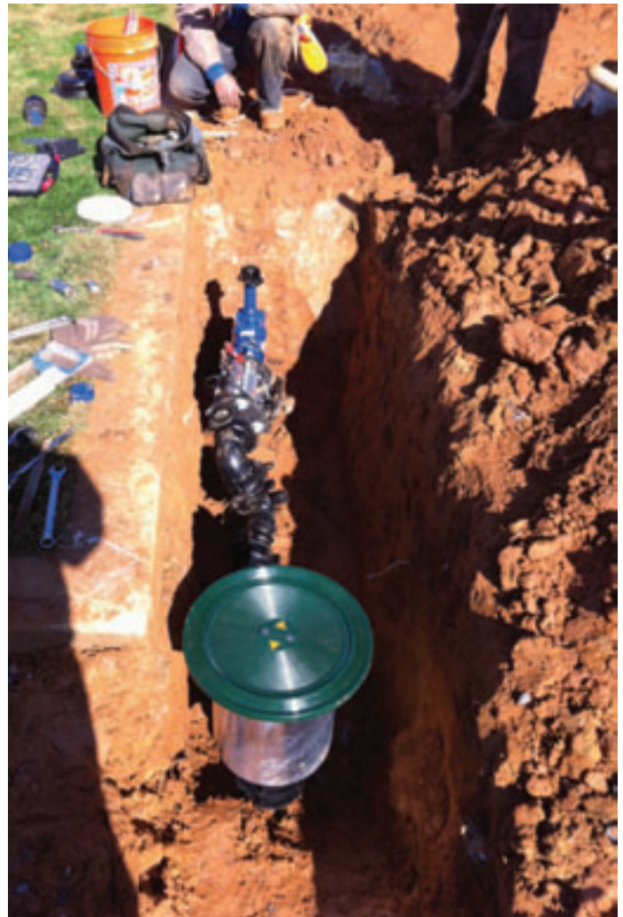
>> Above: UNDERHILL TOTAL SOLUTIONS KITS were installed at KSU. The TS Kits are new all-in-one sprinkler assembly packages that include sprinkler hardware and detailed AutoCad illustrations of the site-specific irrigation system.
