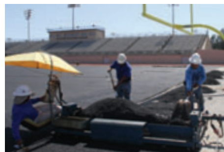
>> Below: AN OPTIONAL ELASTIC LAYER (e-layer) provides additional shock absorption, reduces the cost to replace a field, and drastically improves your turf's lifespan.
