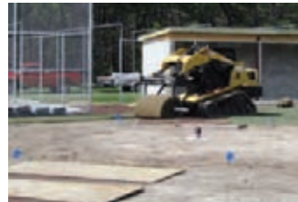
>> Middle Left: "WALK SOFT AND CARRY A BIG RAKE." Low ground pressure equipment was used to install the big roll bluegrass sod.
