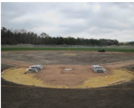
>> Above left: CLAY BRICKS were installed in the pitcher's mound and home plate.
