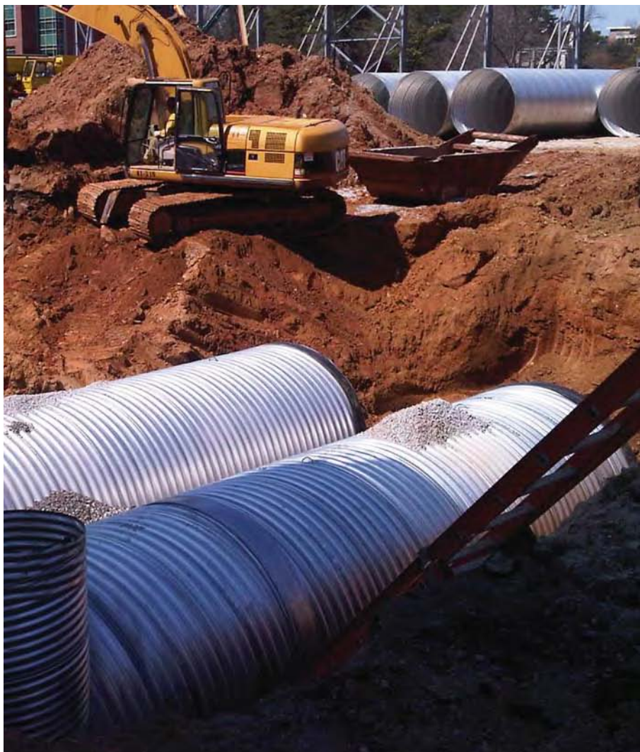
>> A CISTERN being installed under the southwest corner of the natural turf practice field.
