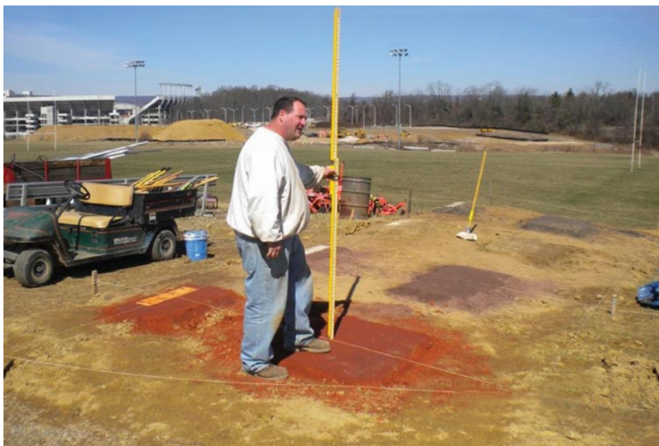
» CHAD KROPFF checking elevation of landing areas
