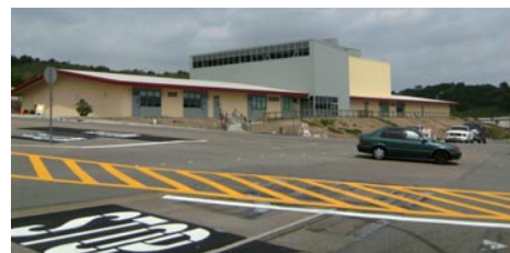
>>THE NEW AGRICULTURE SCIENCE BUILDING at Mt. San Antonio College, Walnut, CA.
