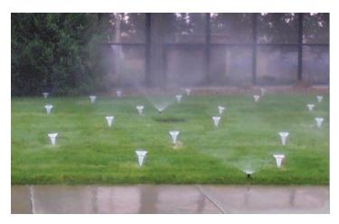
landscaping. Many controllers have special features to allow for more efficient scheduling of the runtimes for the zones. Cycle and soak help save water and prevent runoff, especially if there is a clay soil and/ or slope that are being irrigated.
