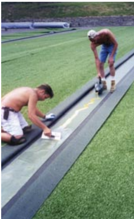
» ADHESIVE being applied to seaming tape with a kneel-down trowel.
