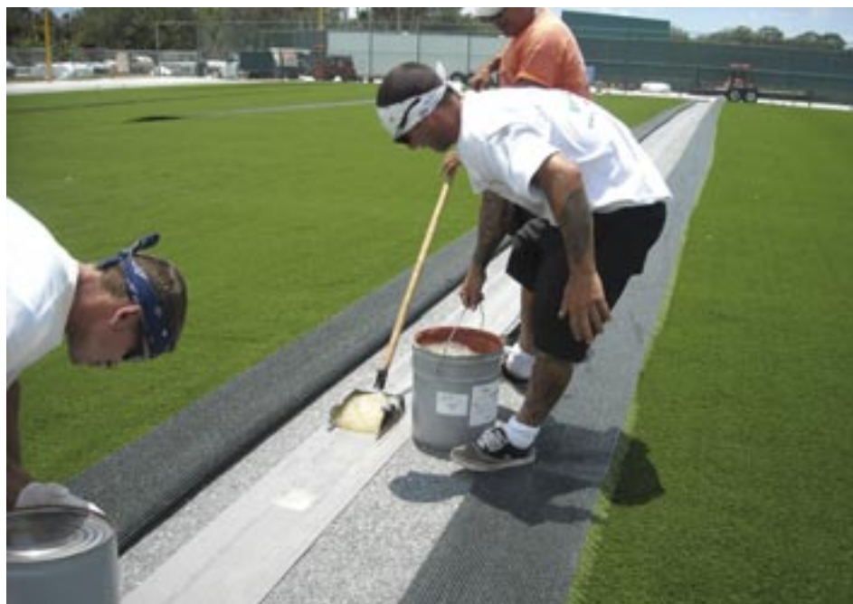
» ADHESIVE being applied to seaming tape with a stand-up trowel.
