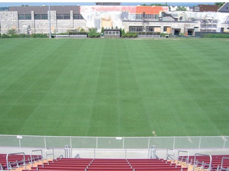
>> Above: TWO MONTHS after sprigging, at the beginning of the fall playing season. Notice that the drainage lines are completely covered with bermudagrass and are still distinguishable. Other than looking a little odd aesthetically, the field functioned very well as a two grass system during the first year. The field was successfully converted to 100% bermudagrass the following summer.
