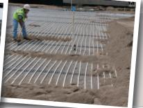
Target Field would then become one of the only MLB stadiums to have a state of the art **hydronic heating system** which was designed to accommodate the seasonal shading of the field. have to removed and disposed off site. Next, 18 inches of select fill was to be installed, compacted, and laser graded. Additionally, it was also tested and approved to meet the stringent specifications of the field design.
