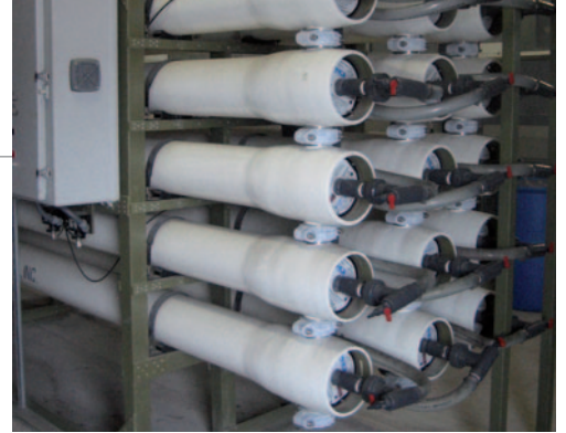
Reverse osmosis systems produce clean water through permeable membranes in a bank of cylinders.
