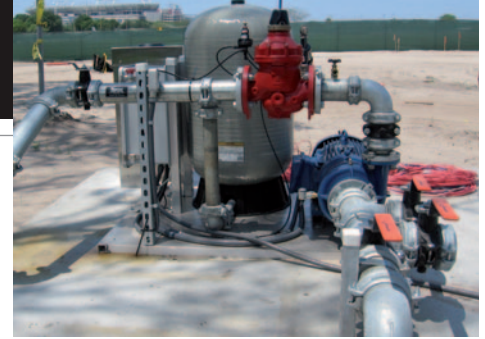
This is signal start, suction lift pump station pulling surface water from a canal adjacent to new football practice fields.
