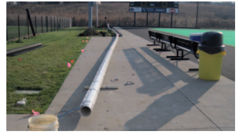
➤ 160-FOOT MAINLINE glued for directional bore under sidelines.
