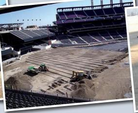
Underneath the field is a network of HDPE pipe that enables Bill Deacon, head groundskeeper, to create a vacuum to remove standing water or force cool or warm air into the root system of the natural grass.
