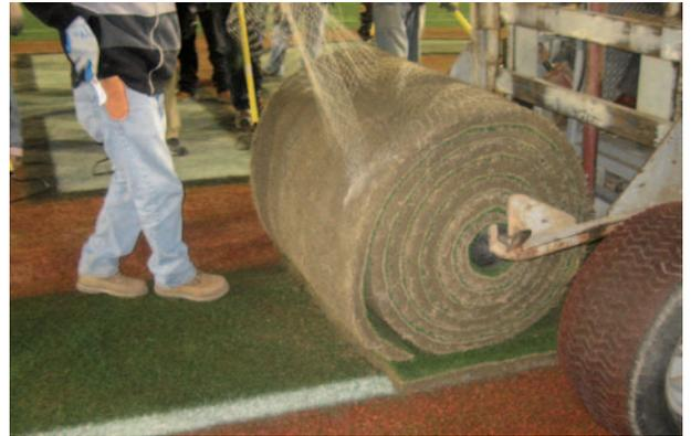
Schnell called Dan Almond to help him map out this daunting mission, and assembled a team to pull it off. Just Moving Dirt was contracted to remove the two sod layers totaling 3 inches, and another 6 inches of the old soil medium. GreenOne Industries installed the new drain matrix (their QwikDrain system). West Coast Sand and Gravel provided the new 6-inch, straight sand growing medium that topped the new
