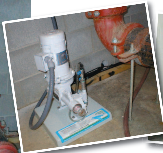
» Left: THE OVERALL VIEW of the fertigation system, controller and connections. » Middle: THE MODEL L 1000 INJECTOR PUMP in the pump room for the complex. » Right: THE 300-GALLON TANK in shop area, with the hose connection through the wall to the injector. The shop area was selected since it has easy access for the fertilizer delivery.
