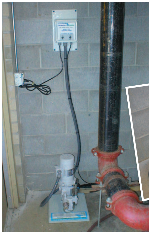
» Left: THE OVERALL VIEW of the fertigation system, controller and connections. » Middle: THE MODEL L 1000 INJECTOR PUMP in the pump room for the complex. » Right: THE 300-GALLON TANK in shop area, with the hose connection through the wall to the injector. The shop area was selected since it has easy access for the fertilizer delivery.
