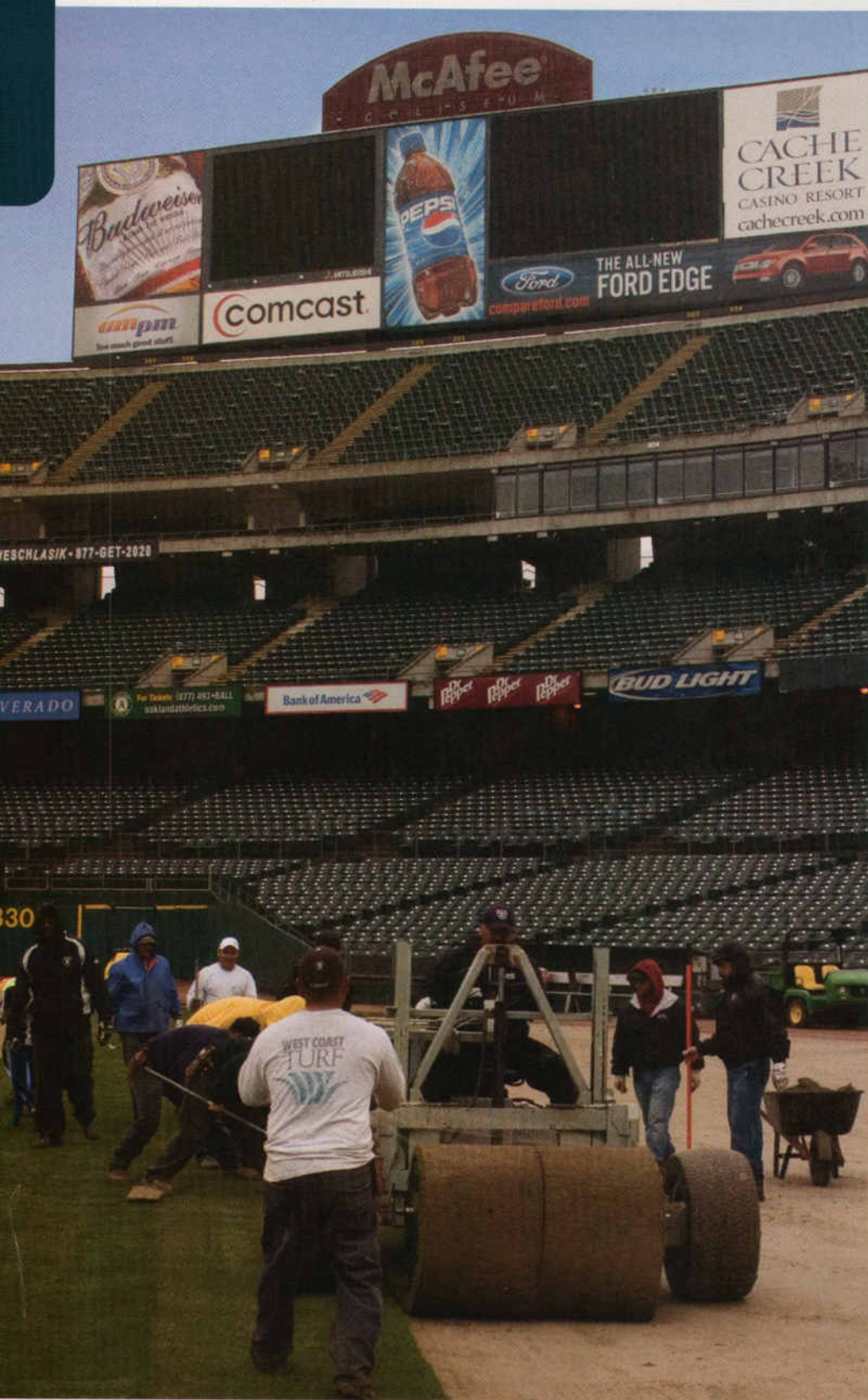
West Coast Turf crew installs big rolls of certified TifSport bermudagrass at McAfee Coliseum in Oakland, home of the Athletics and Raiders.
