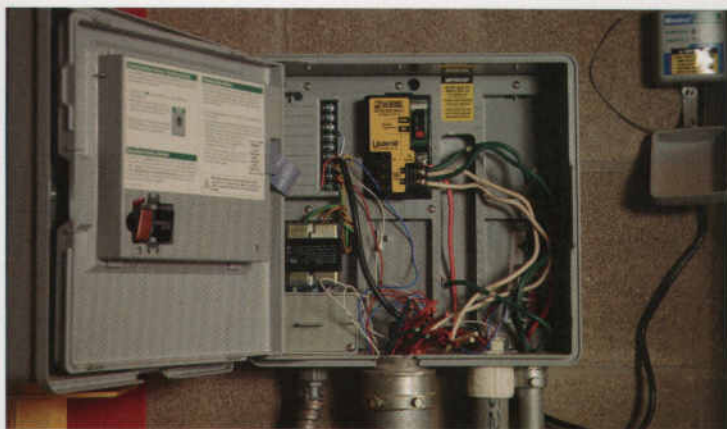
Hunter ICC is set up for operation with two-wire decoder module, which directs all 13 stations.
