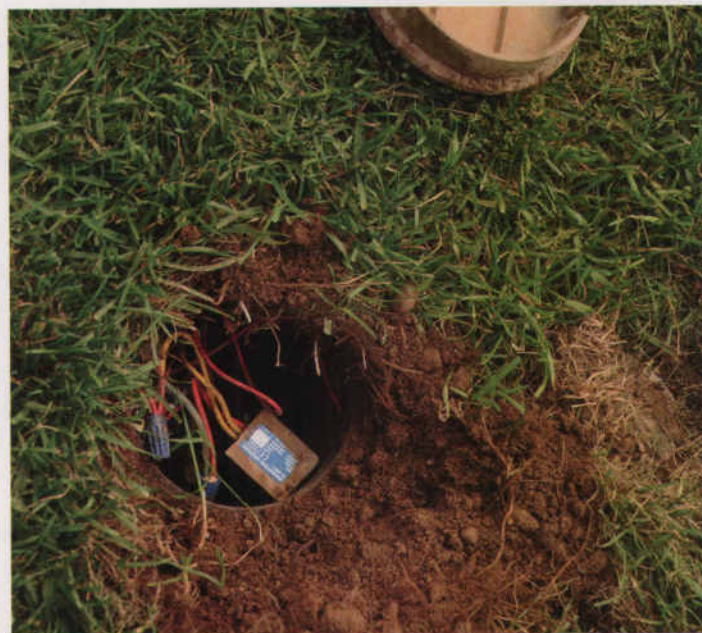
Underhill decoders are attached to every valve and irrigation programming is relayed to each valve over the two-wire system.
