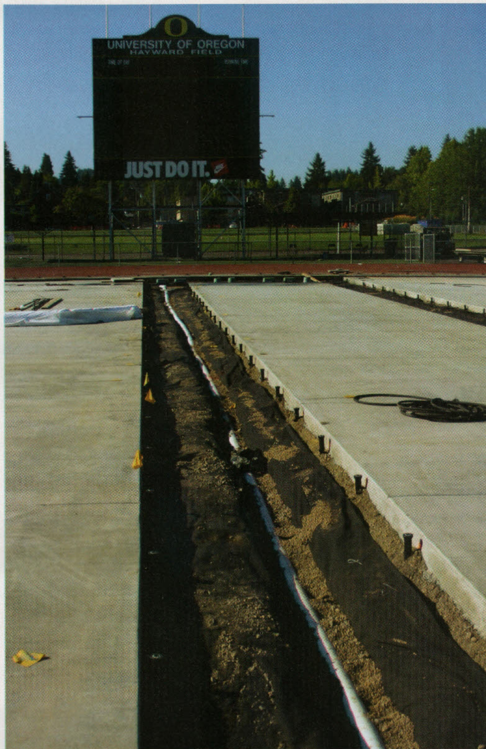
Irrigation and drainage installed in one of the narrow lawn strips. Rexius
