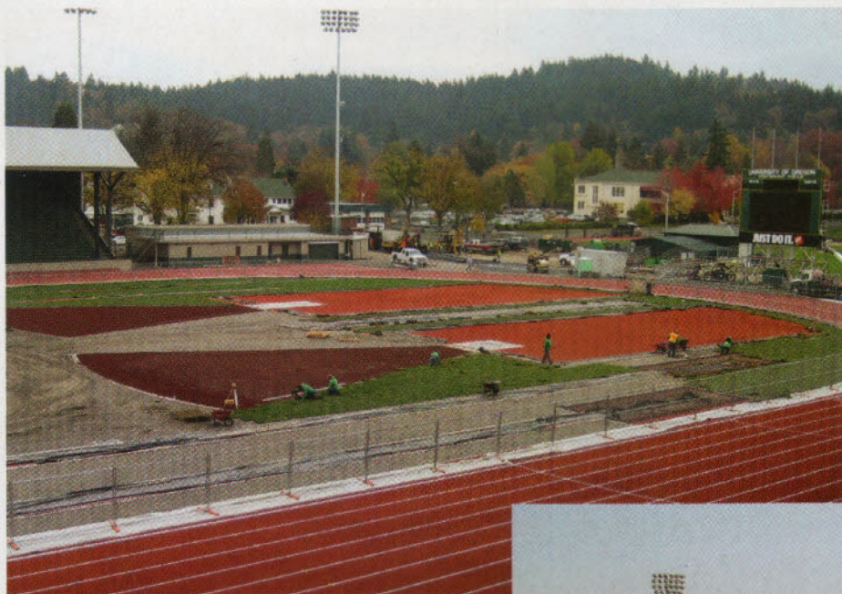
The sod installation. CMGS Landscape Architects
