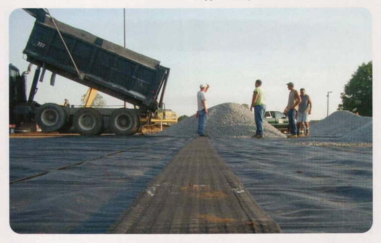
Our design is a "flat" pipe design that has over 70% open inflow space vs. 3% for round pipe. This relates directly to how fast the water can get into the pipe and drain the field. No reservoir is needed to hold the water and feed the pipe.
