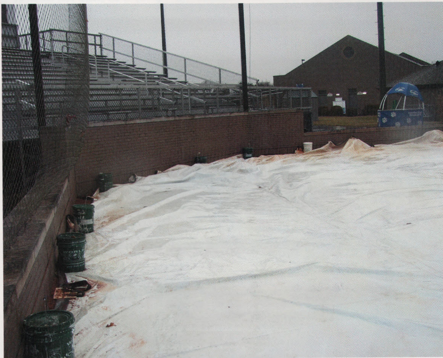
Sand buckets are easier to carry, stack, will not hold water, and will last longer than sandbags.
