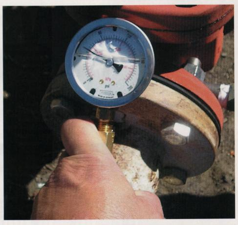
system is equipped with a backflow device, remove any water trapped in the ball valves and testcocks by opening and closing them several times by hand. When fully open or fully closed, ball valves and testcocks have a tendency to trap water between the ball and the housing, so leave them open at a 45 degree position to prevent cracking during a freeze.
