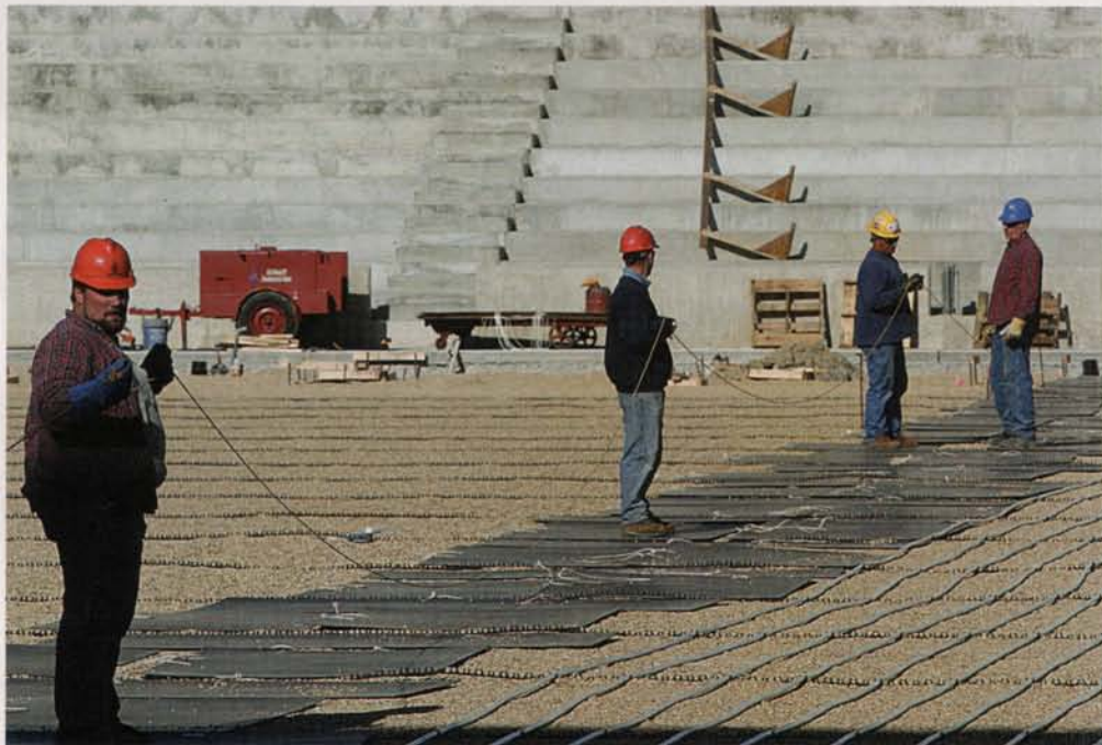
To prevent dimpling of surface with shoe prints, Althoff mechanics stood on sheets of Masonite while working on the field surface.
