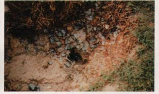
noticed no water movement into the gravel surrounding the socked pipe. I then scratched through the gravel to find the pipe, still no water movement; I then decided to cut the fabric and only then did the water create a vortex that would be the envy of the "Tidy Bowl Man."
