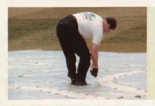
A crew member (left) marks a one-piece, 6 mil poly stencil's color-coded half moon cutouts. When the stencil is removed, the crew (right) connects the dots and fills in with the proper color spray paint.
