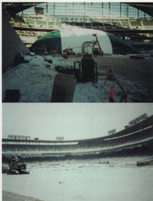
One of Bossard's most challenging stadium projects was Miller Park in Milwaukee. With over a foot of snow on the field and frozen turf, specially designed heating tents had to be brought in to house the 2-million BTU heaters for 12 days to install the irrigation system and the turf.
