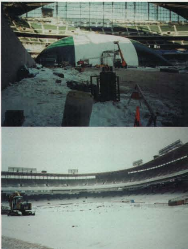
One of Bossard's most challenging stadium projects was Miller Park in Milwaukee. With over a foot of snow on the field and frozen turf, specially designed heating tents had to be brought in to house the 2-million BTU heaters for 12 days to install the irrigation system and the turf.
