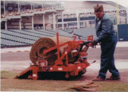
INSTALLED CLEVELAND INDIANS IN 42" AND 48" ROLLS
