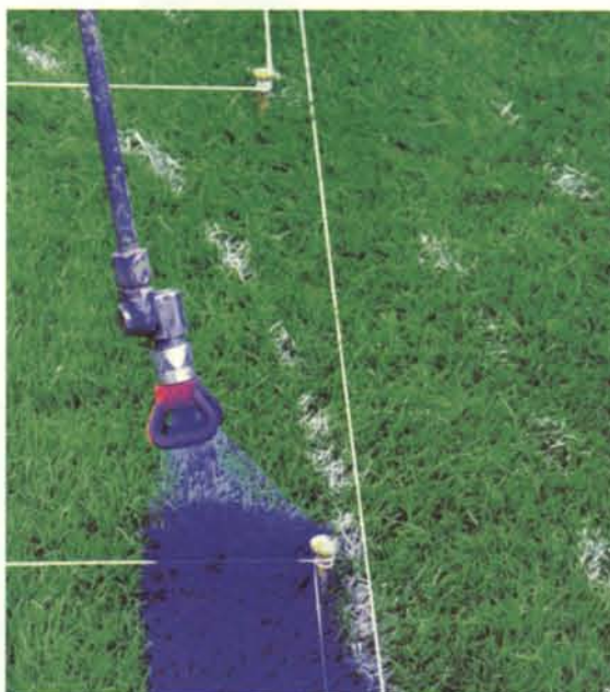
Paint should be applied at a recommended spread rate by spray, brush or roller.
