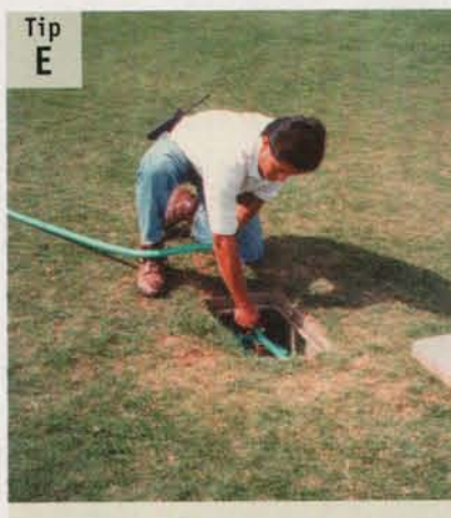
Install a large valve box positioned behind the pitcher's mound to hold watering hose. This avoids carrying the hose in and out daily.
