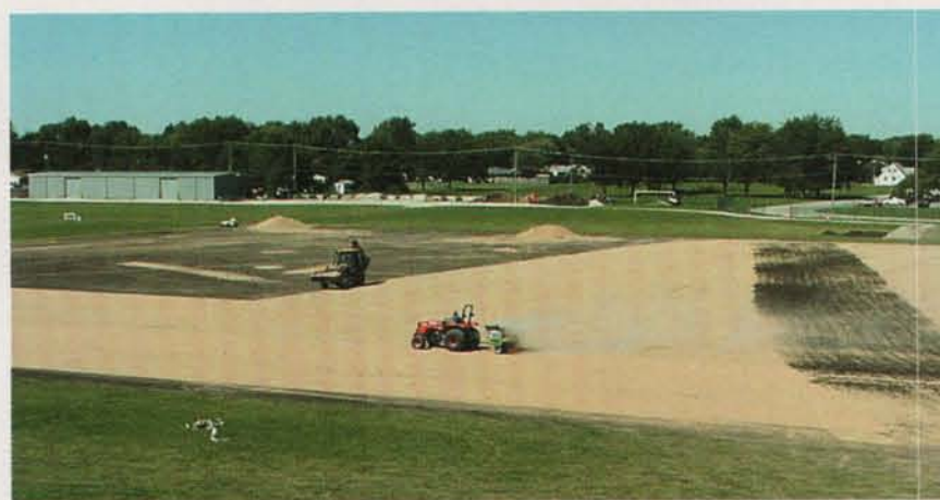
In preparation for the Chicago Bears' training camp, Olivet Nazarene University hustled last year to complete a $1.5 million renovation project, which included laying new sod, installing an underground irrigation system and adding TURFACE MVP to the fields.
