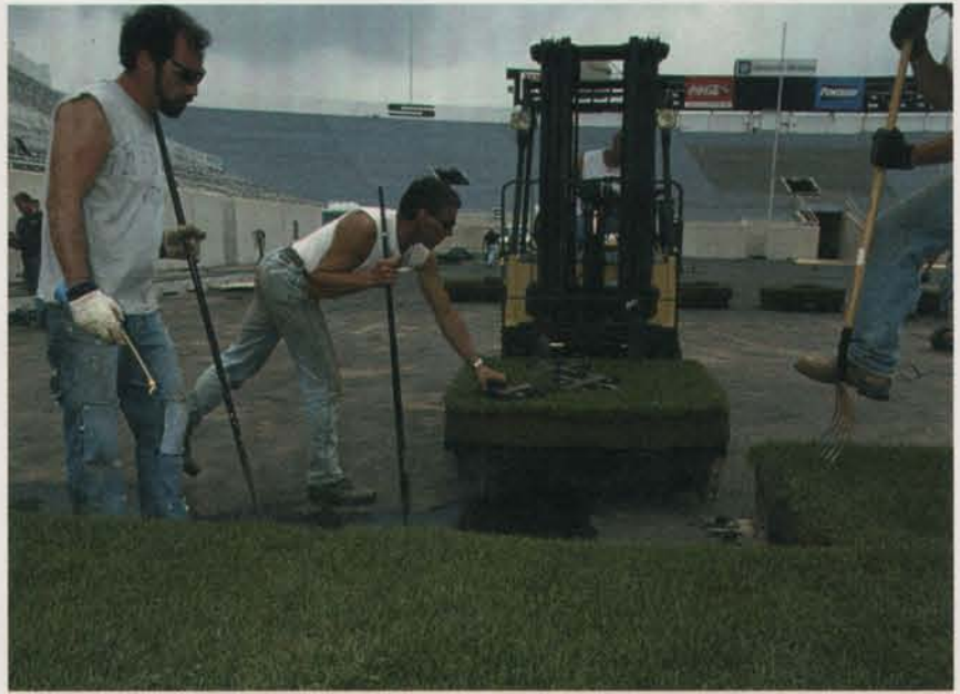
The modules were placed in the same order that they occupied at the Hancock Turf Center so that the edges and seams fit back together tightly.
