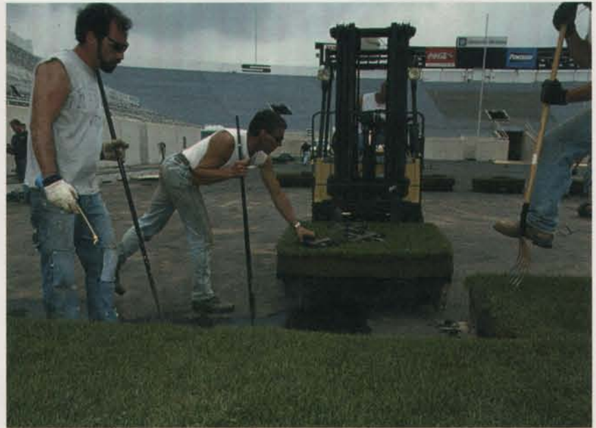
The modules were placed in the same order that they occupied at the Hancock Turf Center so that the edges and seams fit back together tightly.
