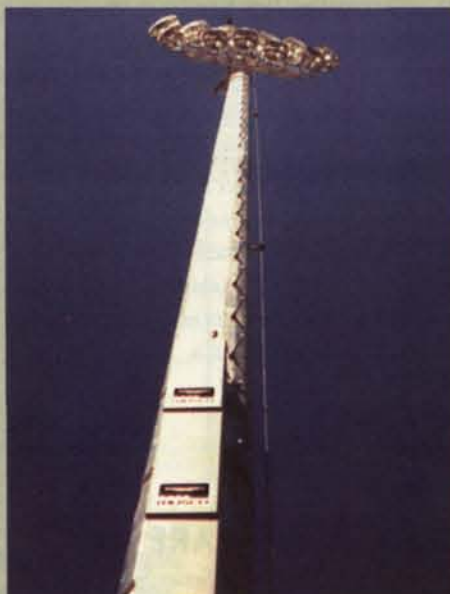
Illinois School District 211 was able to strike a 10-year agreement with Sprint in which Sprint paid for four light towers as well as any electric bills associated with the use of those towers.
