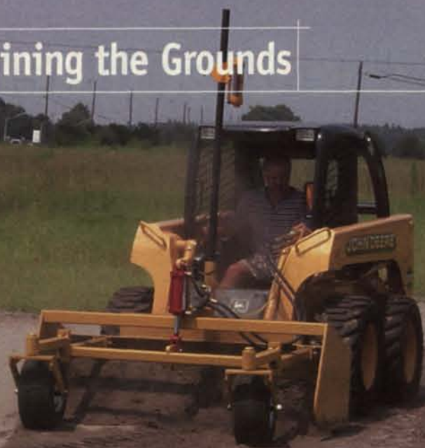
A grading tractor equipped with a laser controlled box blade can easily grade to within 1/4 of an inch.
