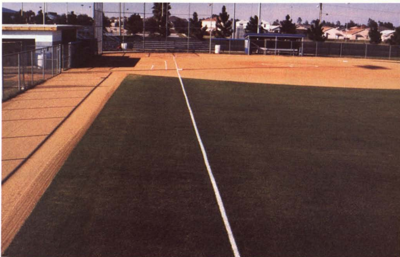
County personnel used laser-grading equipment to establish a one percent slope toward the foul lines and toward the backstop.
