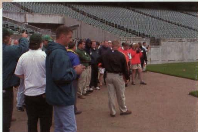
Doug Bradley describes the new Astrograss (a product of S.W. Recreational) system he is installing at Paul Brown Stadium. In this system, grass is grown on a mat with grass fibers and a 50% biodegradable backing. The installation was about 3/4 complete.
