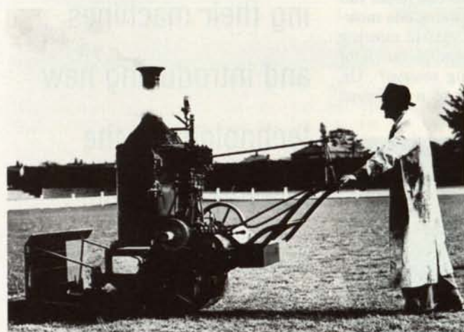
A Leyland steam-powered mower designed for sports turf.
