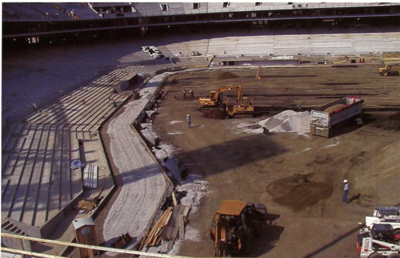
A solid foundation is important to quality turf. Here, workers prepare the soil mixture on which the sod will be laid.
