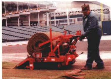
INSTALLED CLEVELAND INDIANS IN 42" AND 48" ROLLS
