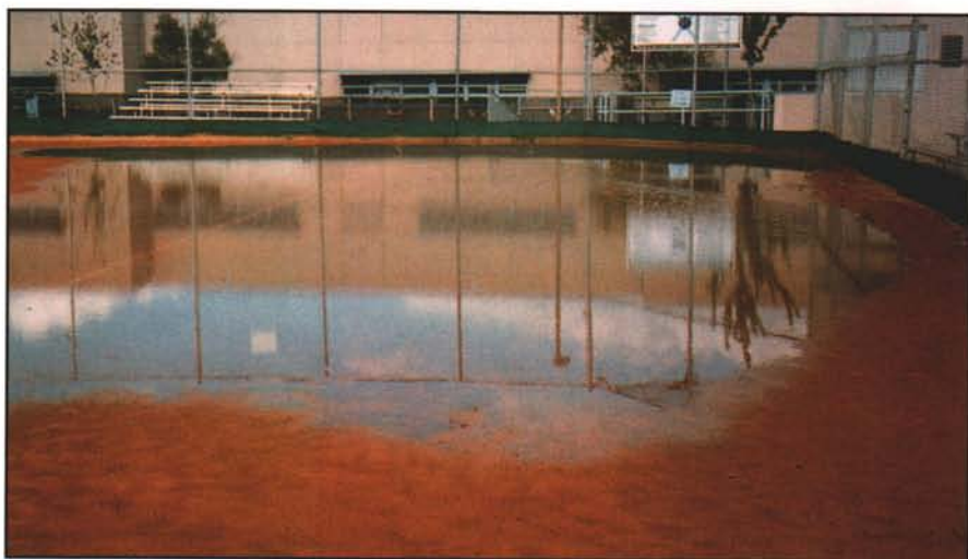
Heavy traffic on this baseball field has led to serious drainage problems.
