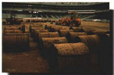
The weight of thick-cut sod, not deep, established roots, make it immediately usable for play. Courtesy: Tony Koski
