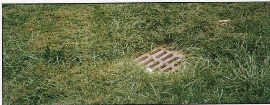
A hidden sewer cap on an athletic field can lead to a series injury and potential lawsuits.
