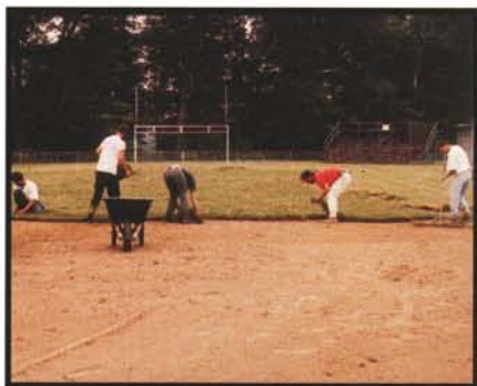
Strip sodding on a field in north-east Ohio. Courtesy: Jim Puhalla
