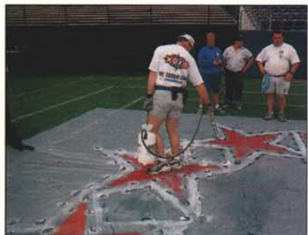
The crew used hand-held compression sprayers for fine detail work on the field's logos. Courtesy: Steve Wightman.
