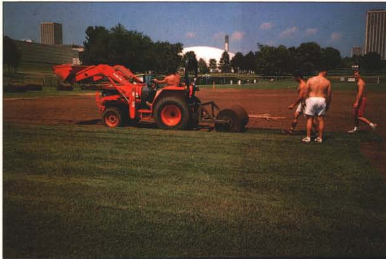
The team rolled out 270,000 feet of sod, four feet at a time. Courtesy: Toro.
