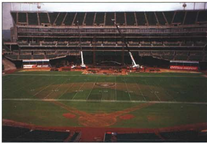
As Nor-Cal's meeting progressed, so did construction of the six-story-high stage for the Rolling Stones tour.
