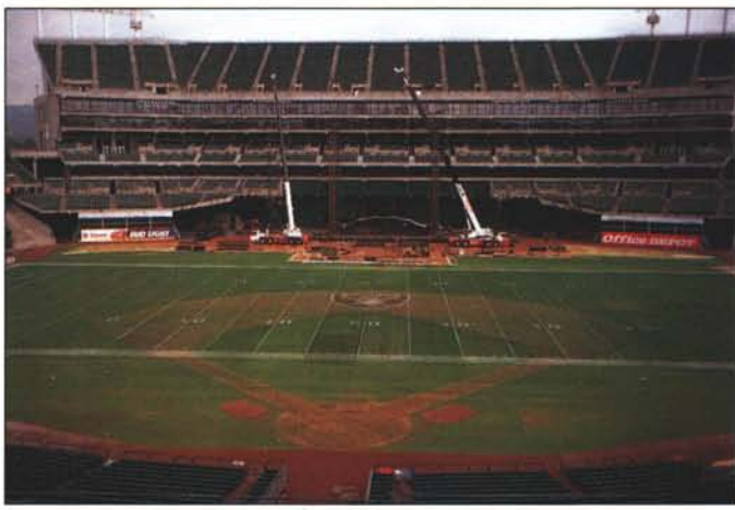
As Nor-Cal's meeting progressed, so did construction of the six-story-high stage for the Rolling Stones tour.
