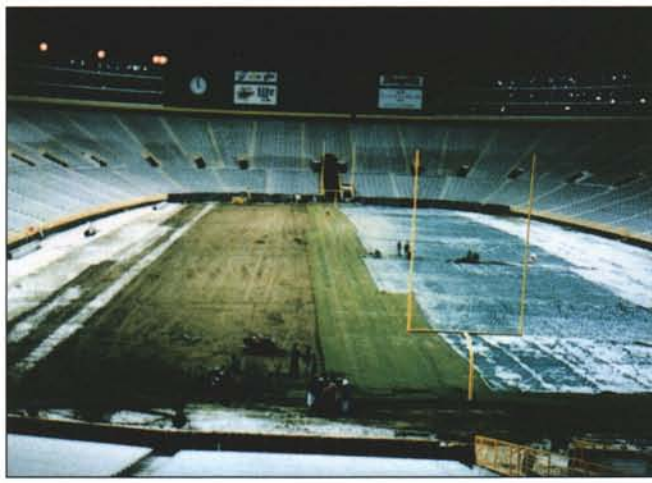
By late Wednesday night, two-thirds of the field was sodded, but a snow storm was yet to come. Frost areas on the perimeter show the failure of the warming cables.
