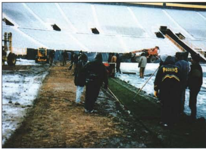
When workers discovered low areas after stripping the old sod, sand was brought in (background left) and spread evenly before the new sod was laid.
