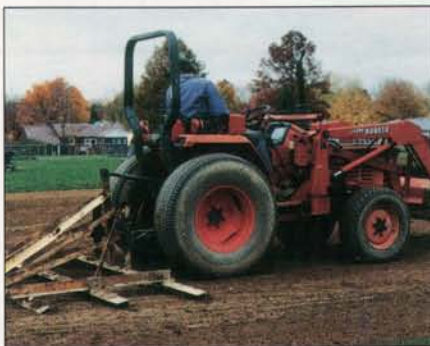
A level bar up to ten feet wide helps get a smooth, consistent surface. This one was easily made in the contractor's shop.
