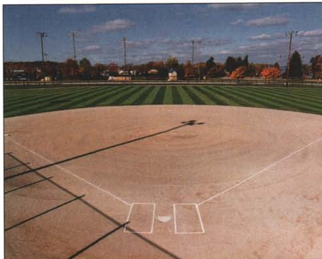
The infield surface is made of crushed limestone screenings, called "stone dust," which is relatively inexpensive. Photo courtesy: Mike Varner.
